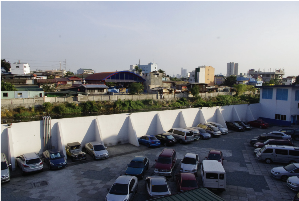
The UERM Medical Center built water walls and flood gates to prevent floodwater from the river from reaching the hospital.
