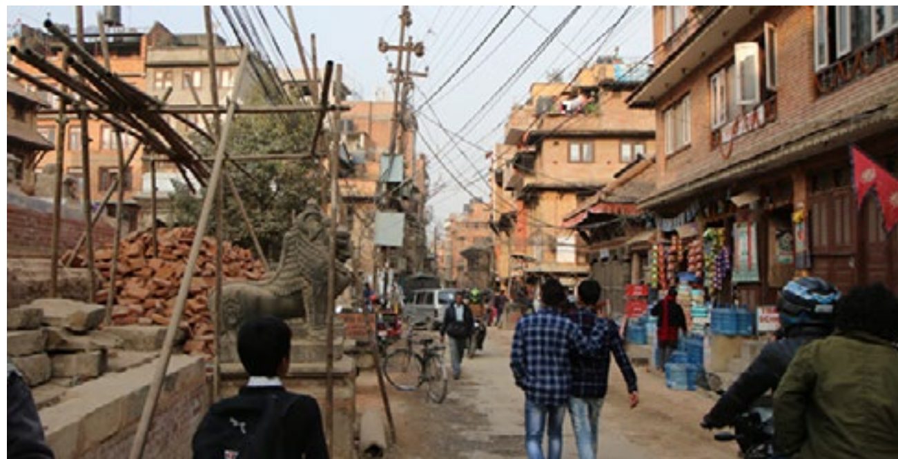
Ongoing earthquake reconstruction work in Nepal. Photo by Vidya Rana.
