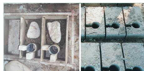
Broken stones from demolished school buildings are filled into molds (left) to make stonecrete blocks (right)
