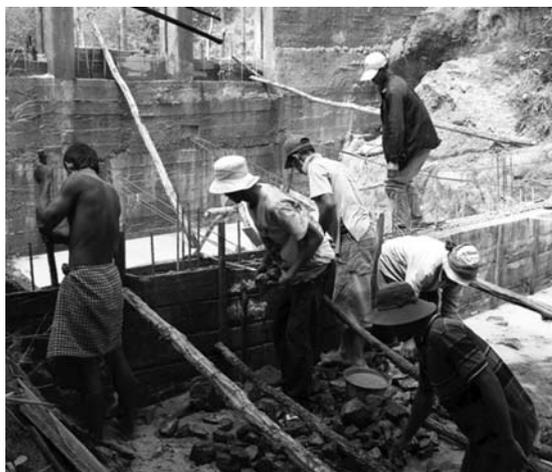
The water gate, located 2 km from the village, down the mountain side, was constructed in February 2008 on the broken end of the dam built in the 1970's. The dam was destroyed by illegal fishermen after the Khmer Rouge period. The gate is 16 m in length, 5 m in height and 4 m in width. The water gate holds the water flow from the upper stream and the mountains and direct it through a small hand dug canal to irrigate the farmers' paddy fields.
