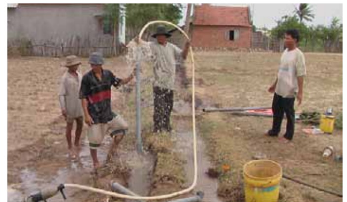
Figure 2. Digging a new well in the coastal area
