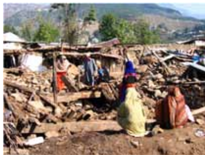
Earthquake damage, Pakistan 2005 © Karl Schuler, IUCN
