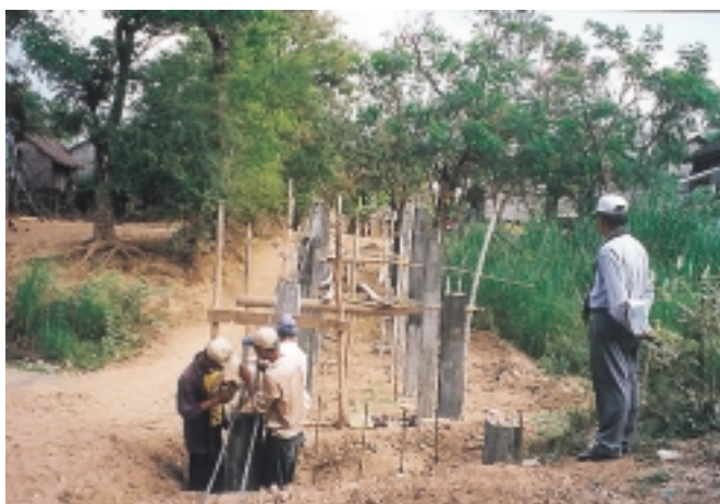
Communities work together to construct a bridge in Prey Veng.
