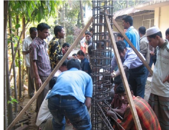
Training for Masons and Bar Binders
