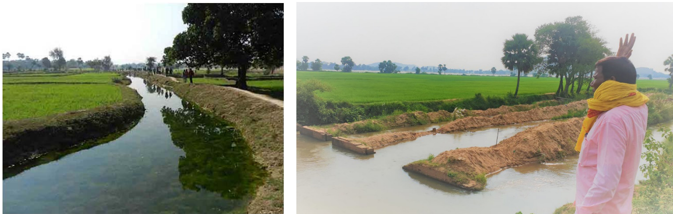
Figure 10: A Pyne conveying water to farms (left source: India Water Portal) and a revived system running full capacity. (right, source: WHH)
