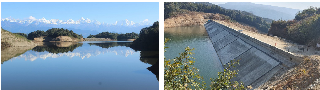
Figure 8: Dhap Dam and reservoir (left) in the head-reaches of Bagmati River and the Concrete Face Rockfill Dam (on right) (Source: DoWRI, GoN).
