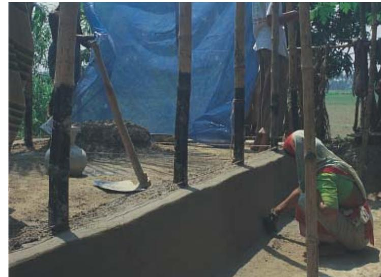
*Fig. 2.4 Painting lower end of bamboo post with bitumen*
