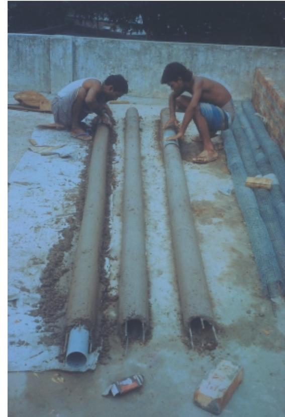
Fig. 5.2 Details of hollow RC post and its production
