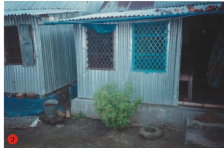
Fig. 2.1 Cement-stabilized earthen plinth
