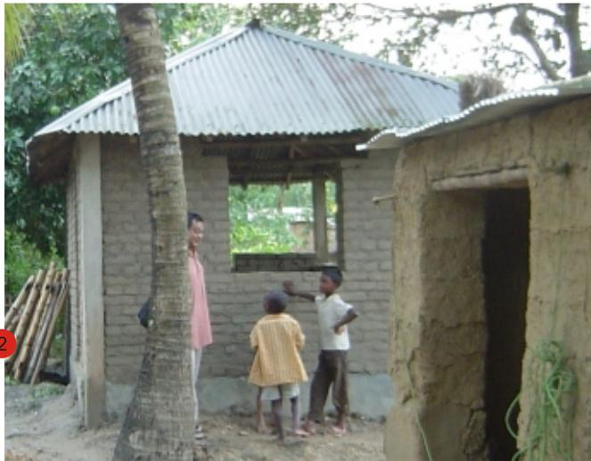
Fig. 4.6 Compressed earth blocks
