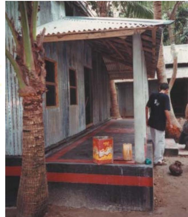
Fig. 2.3 Cement concrete flooring detail and house with cement concrete plinth
