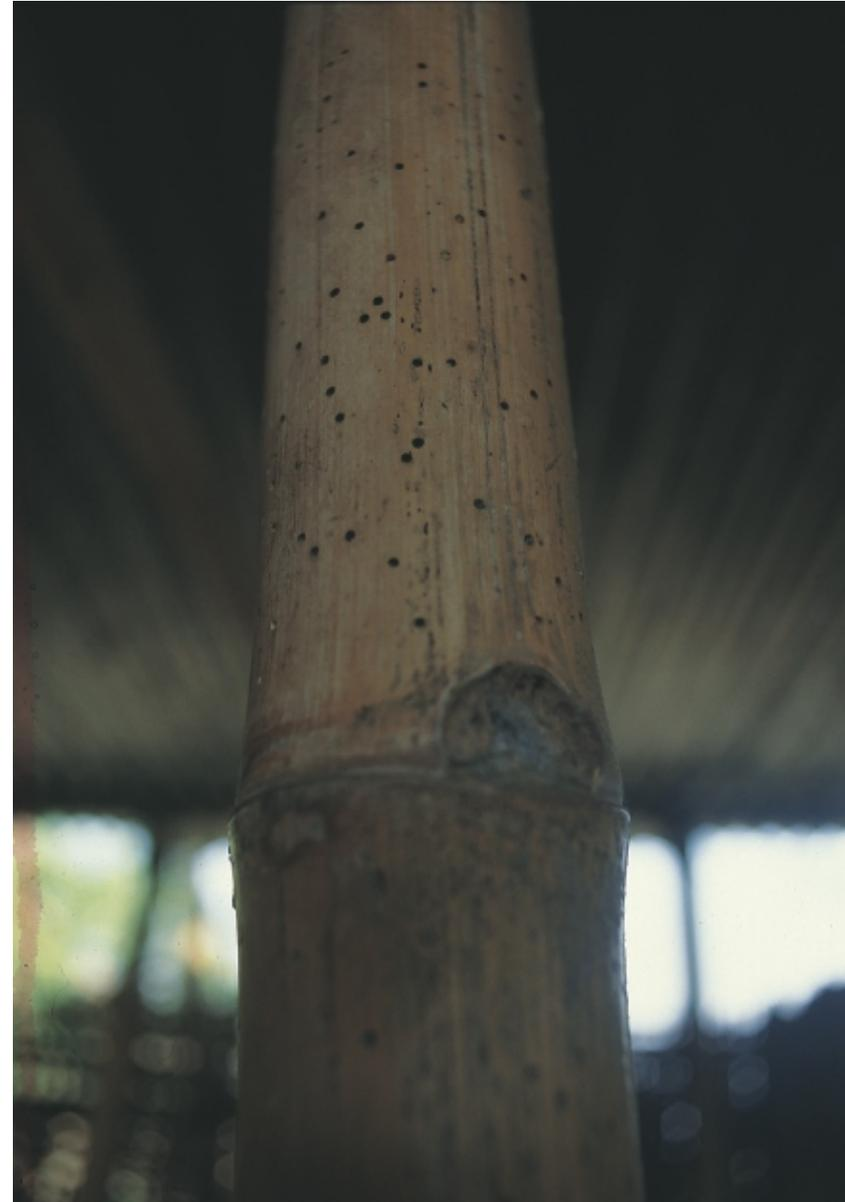
*Fig. 3.1 Bamboo post under insect attack*
