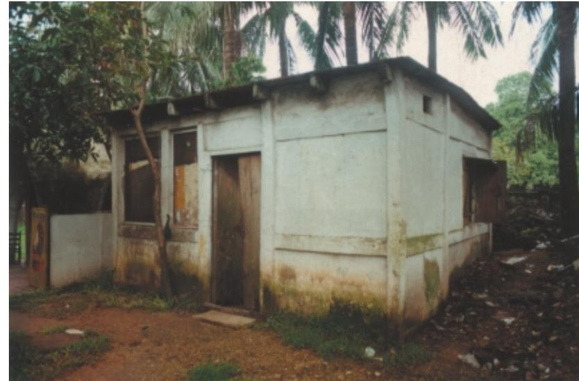
Fig. 5.3 House made of ferrocement wall and roofing panels
