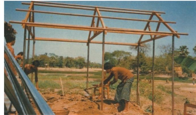
Fig. 5.7 Example of metal structural frame in house design by EDM (from EDM)
