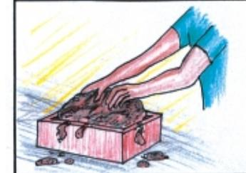
Soil-cement mix to be placed in wooden brick mold and compacted by hand.
