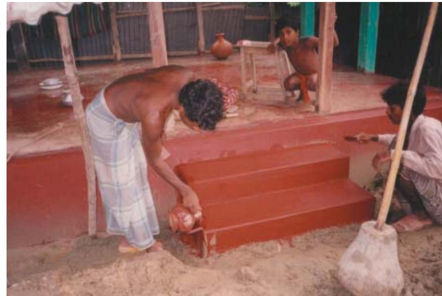
Fig. 2.2 “Dowa-posta” plinth construction
