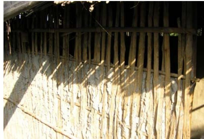
*Fig. 4.2 Wall built in the wattle-and-daub method*
