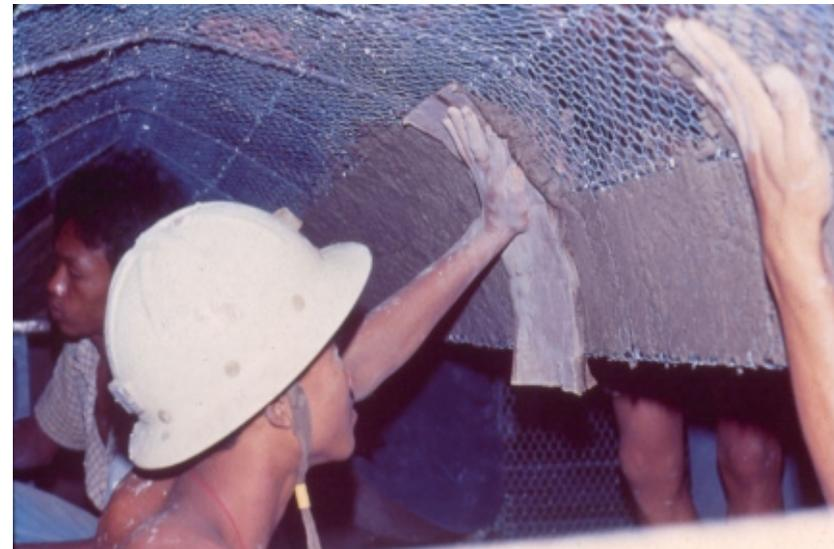
Fig. 5.4 Ferrocement construction process
