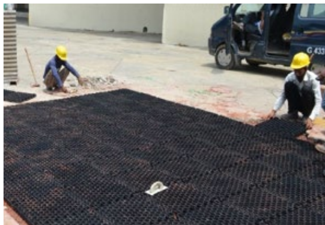
Setting down the GridMats technology over damaged roads (Photo by: PotHole Raja, 2021).
