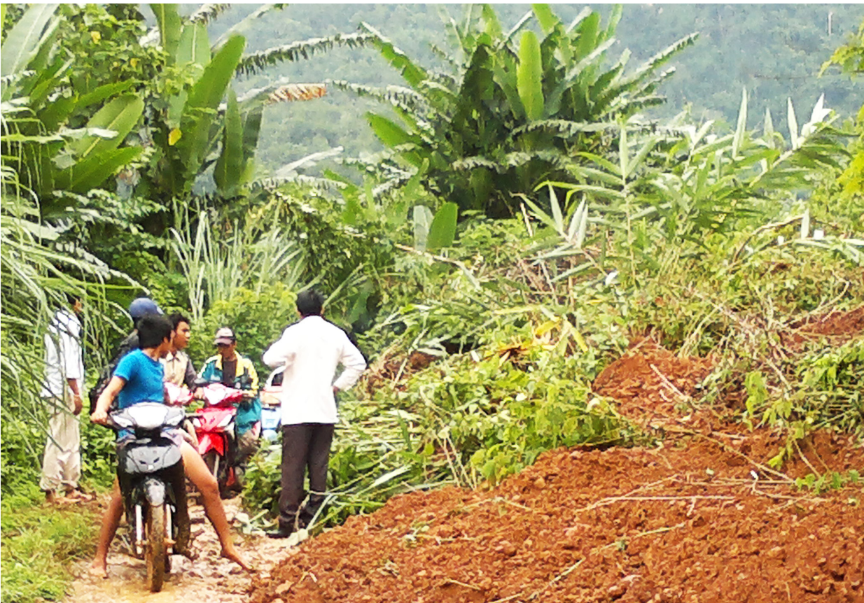
Landslides which affect road networks are a common occurrence
