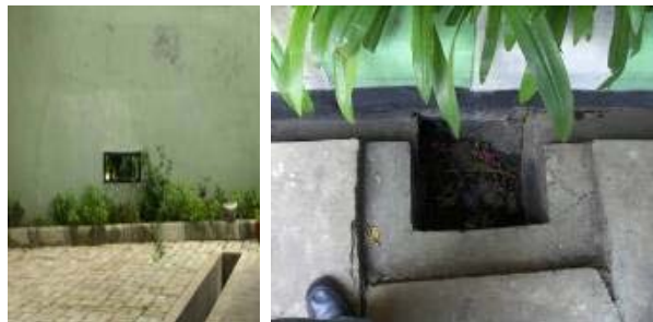
Figure 19 : School DRR Initiatives on : Holes at the wall fences around the school and drainage system connected to Ciliwung River
