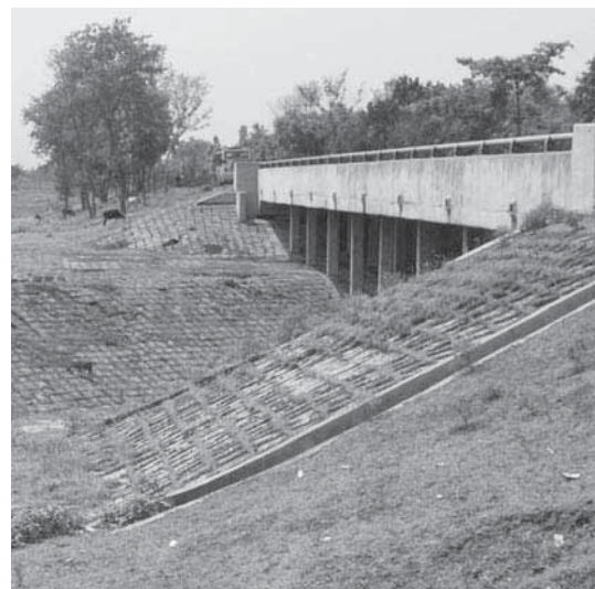
left. Embankment , right. Stabilised embankment and culvert to prevent gullyng
