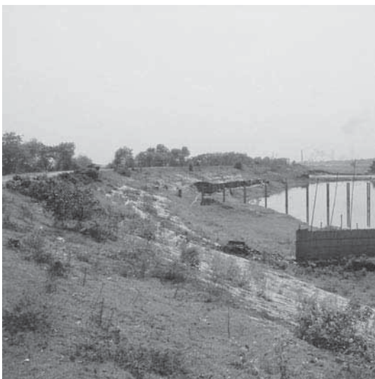
left. Embankment , right. Stabilised embankment and culvert to prevent gullyng
