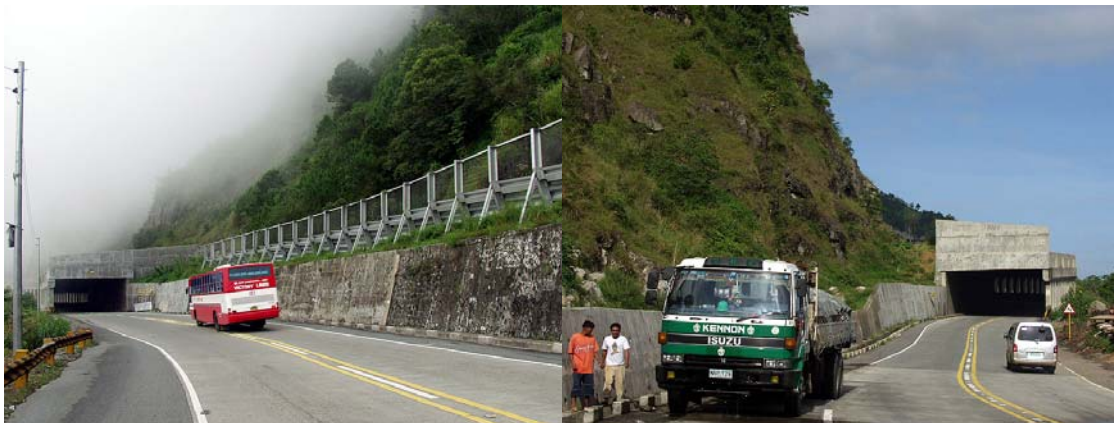
Fig. 13 Rockslide shelter and barrier along the highway leading to Baguio City.
