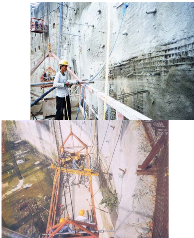
Fig. 12 Soil nailing and rock bolting, RCBC Plaza, Makati City, Metro Manila.
