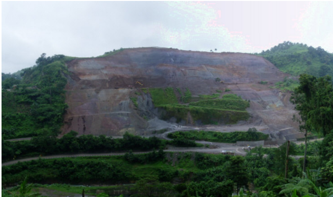
Fig. 8 Benching of slopes in Tongonan, Leyte.
