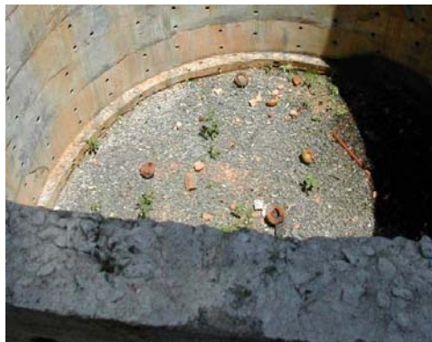
Drainage well at Marangahawela landslide on Colombo-Ratnapura-Wellawaya-Batticaloa Road on 170 th km
