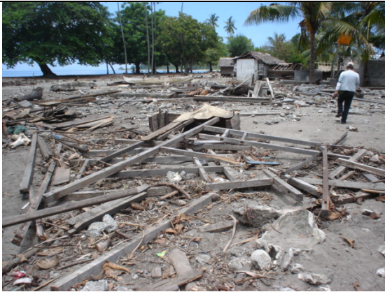
Figure 5. Collapse of housing in Buru Island by earthquake on March 14, 2006 not by tsunami.
