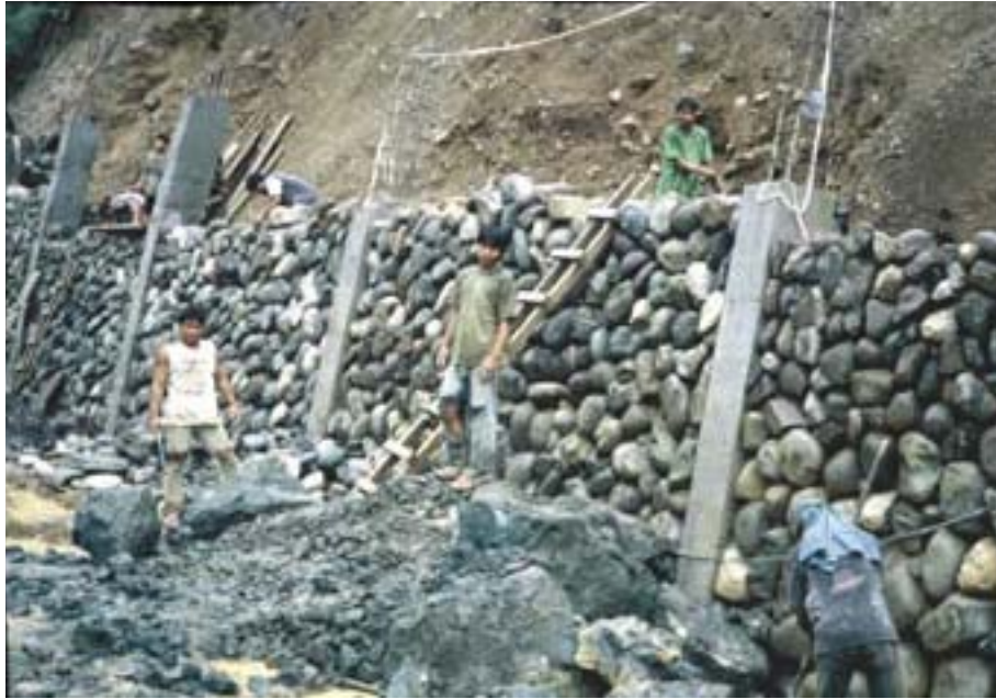
Fig. 10 Grouted Riprap walls along Halsema Highway, northern Philippines.
