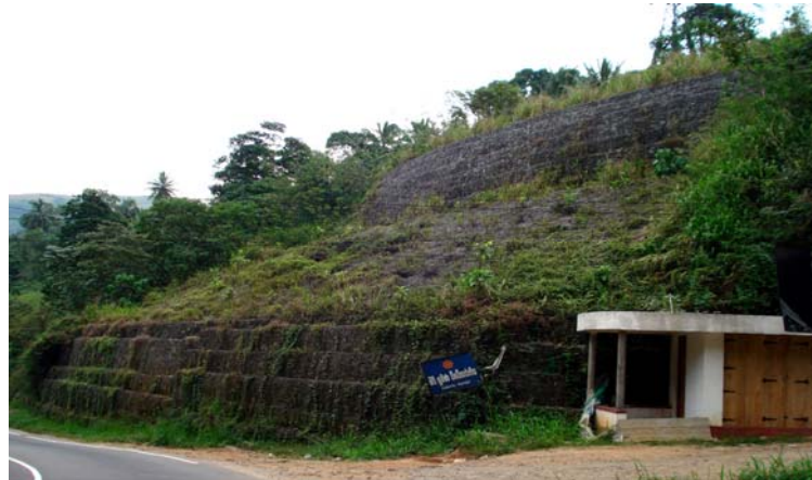
Gabion Construction at Balakaduwa
