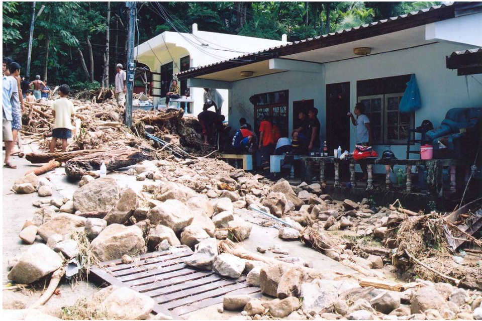
Figure 3-7 Flooding and debris flow on 14/10/2004 at Kalim village.
