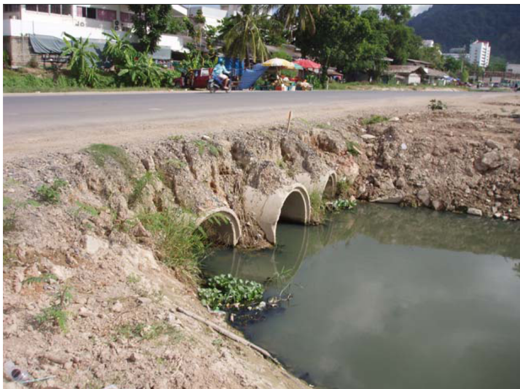
Figure 4-21 Bridge 7 from downstream
