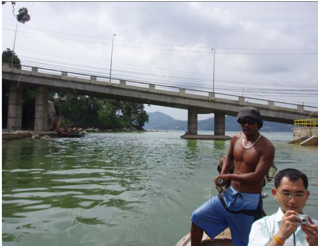
Figure 4-15 Bridge 1 from downstream
