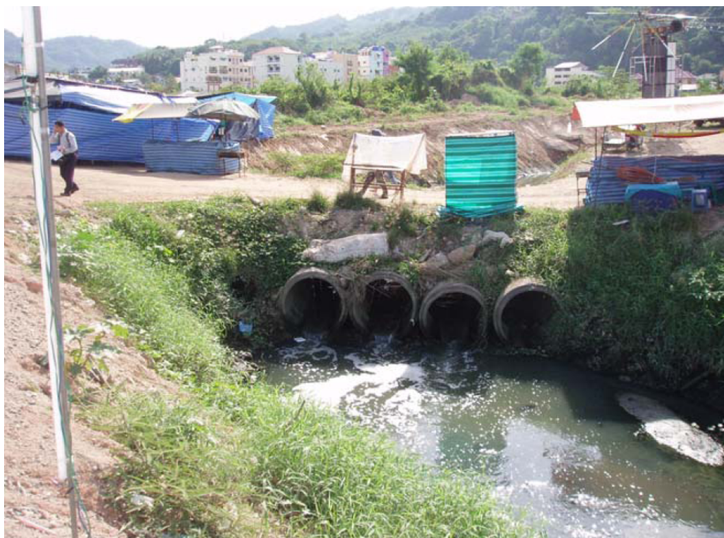
Figure 4-19 Bridge 5 from downstream
