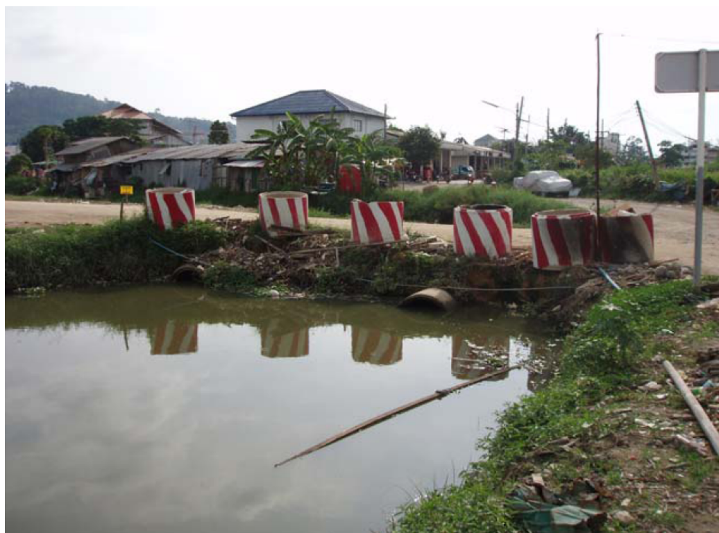
Figure 4-17 Bridge 3 from upstream
