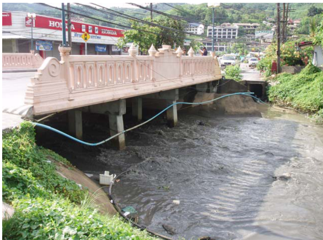
Figure 4-16 Bridge 2 from downstream (taken after rainfall)
