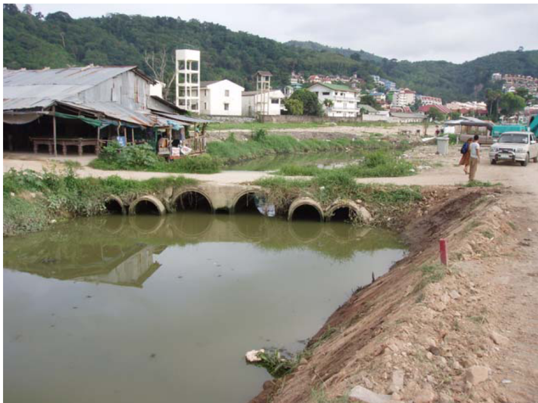
Figure 4-18 Bridge 4 from upstream
