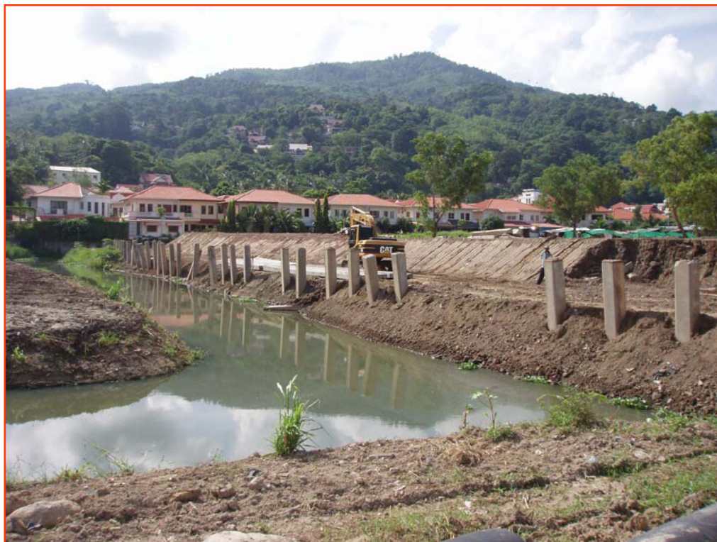
Figure 4-1 Channel construction between bridge 6 and 7 (see later description of bridges/culverts)
