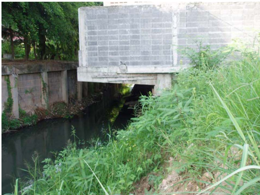
Figure 4-20 Bridge 6 from upstream closure.
