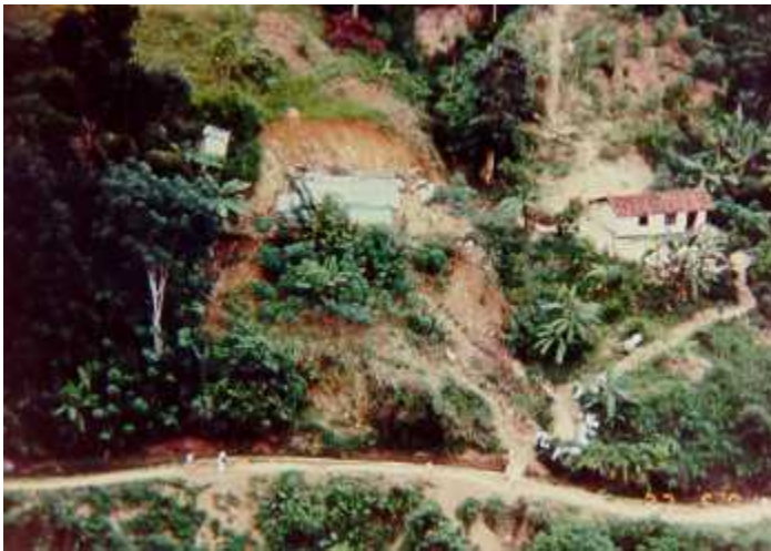
Figure 3. Hap-hazard constructions in Kandy area
