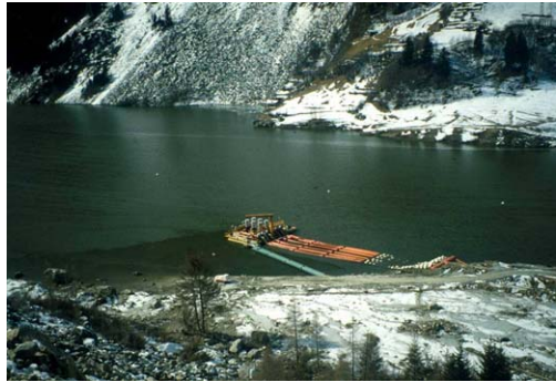
Figure 10 Pumping station Capacity (11m cubic meters/sec)
