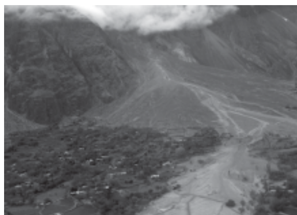
Debris flow hazards increase the vulnerability of the community
