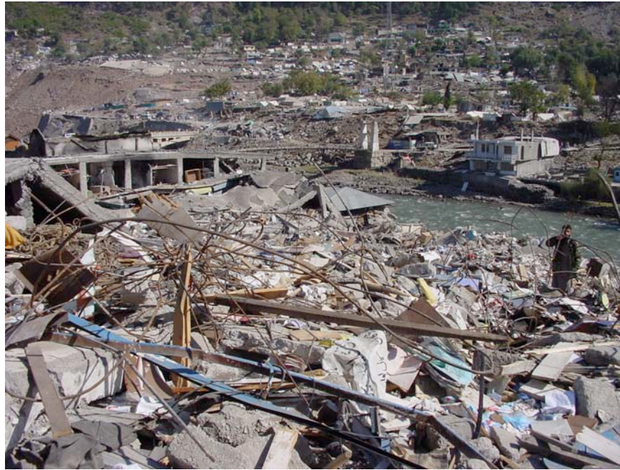
Devastation at Balakot
