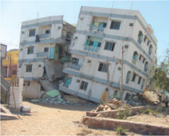
Building collapse during the Gujarat Earthquake, Photo: UNDP website
