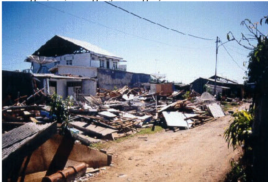
Figure 9 Example of residential damage in Bengkulu City
